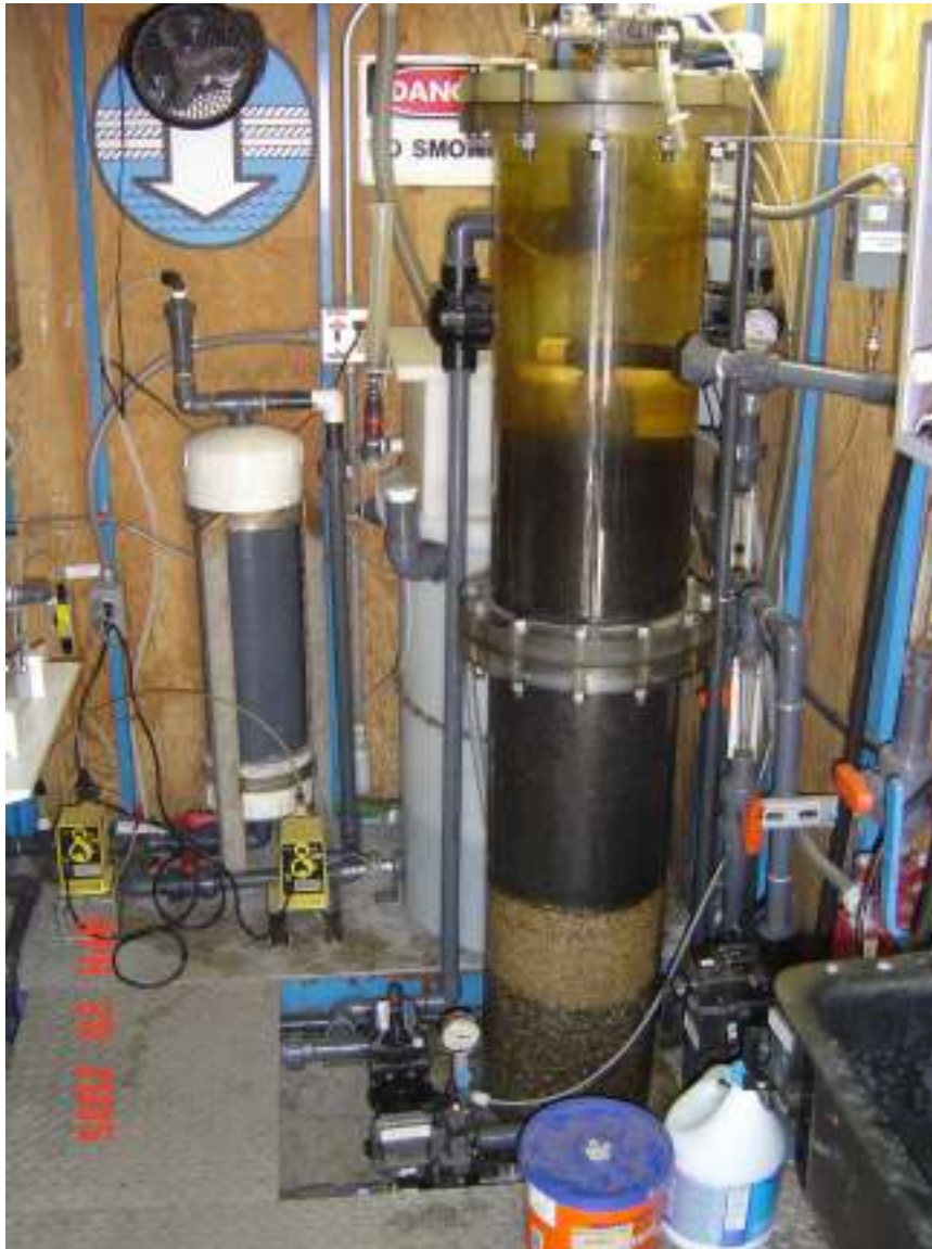
FIGURE 1 INTERIOR VIEW OF TRAILER
